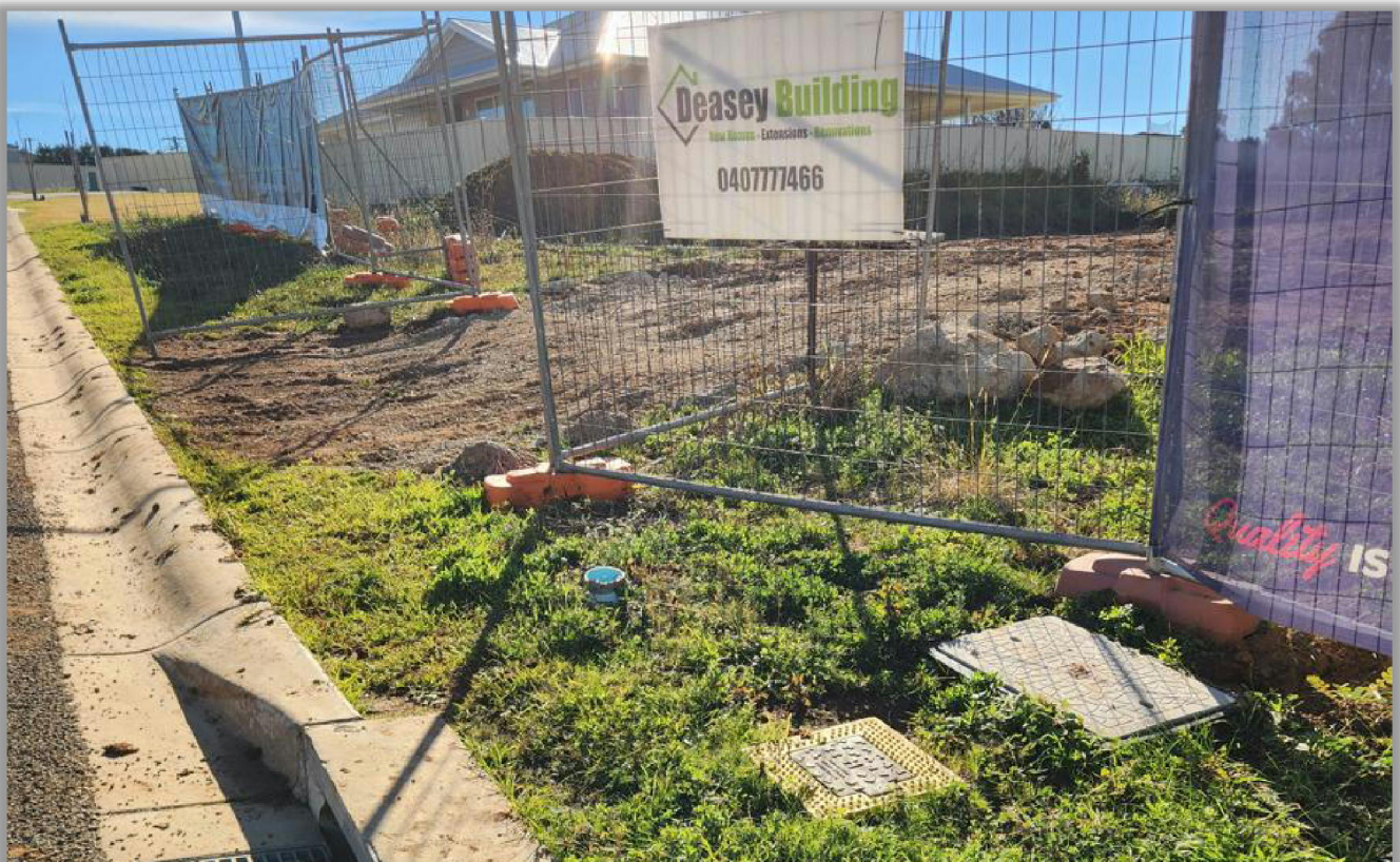
Services at front of site
