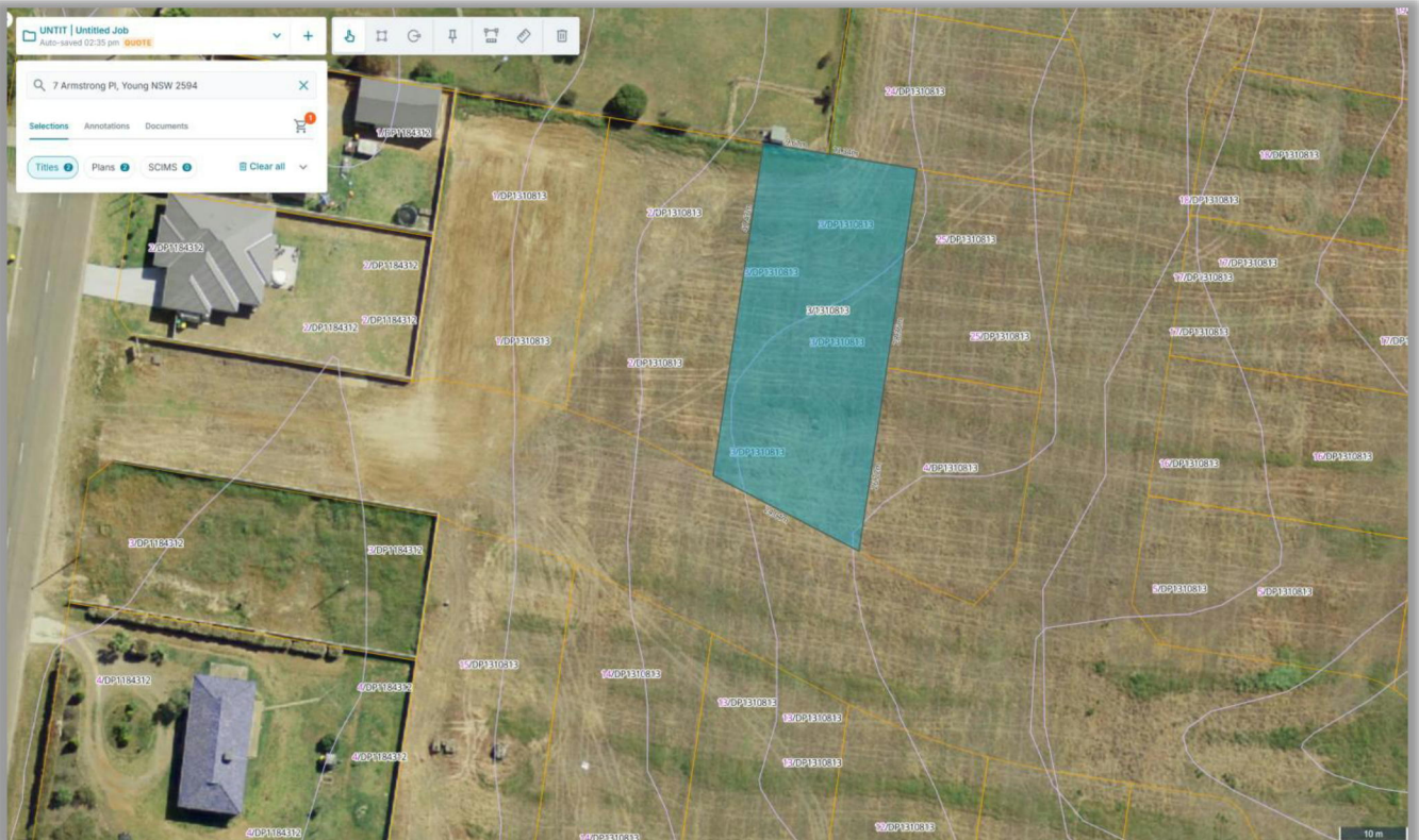
Aerial Image (Source: InfoTrack MapIT) – 200mm contours – NW to SE slope underlying the cut/fill from subdiv stage
