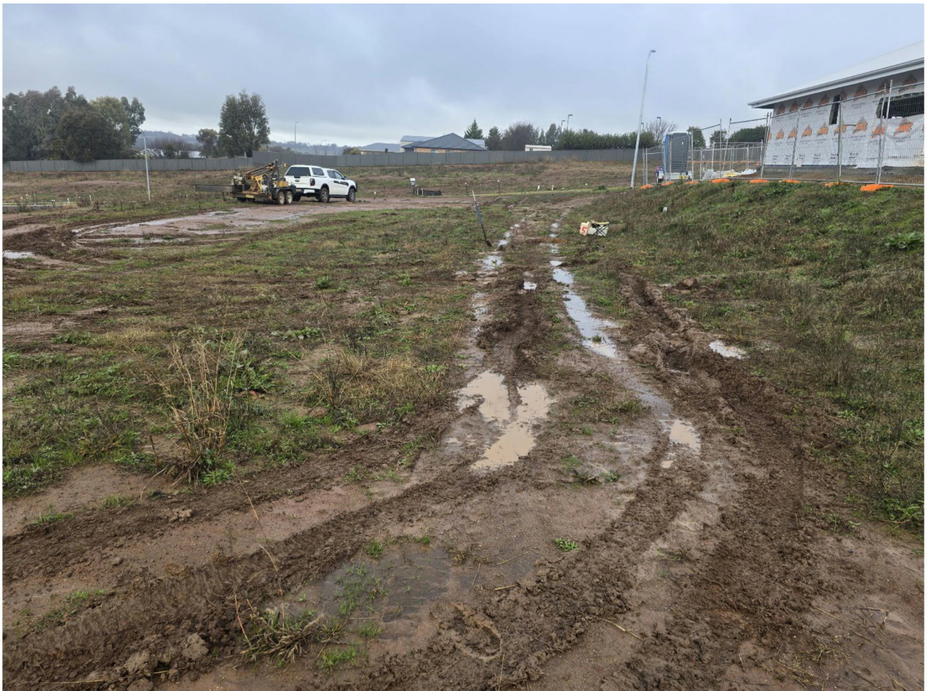
Site Photo – BH1 Looking South (29/07/2025)
